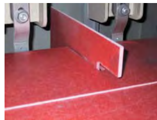
After Cleaning Figure 10
