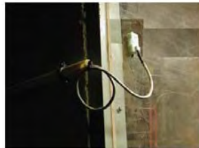
Figure 10. An Arc sensor installed at wall of a cubicle.
