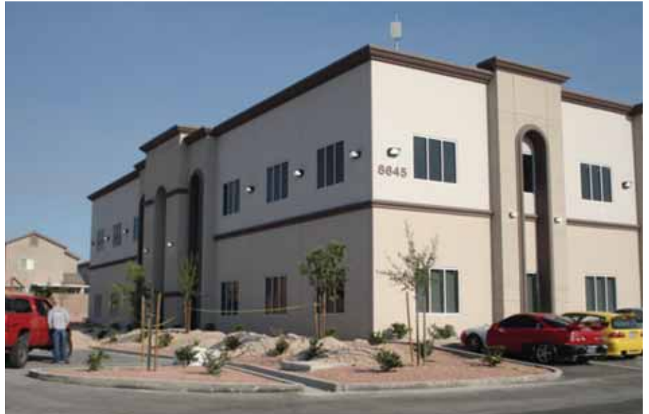
Network Solutions Group gets grounding down to less than 1 ohm with an external grounding system, protecting its data center from the ferocity of Las Vegas thunderstorms.
