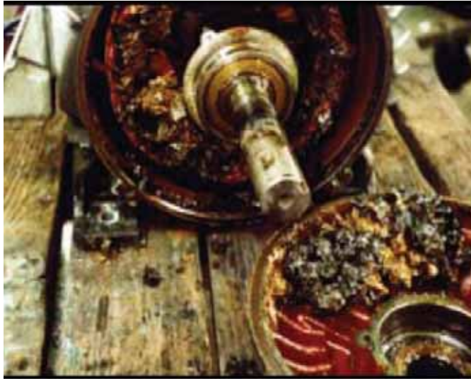
Figure 9. Over-greasing caused the inside of the motors to fill with grease.
