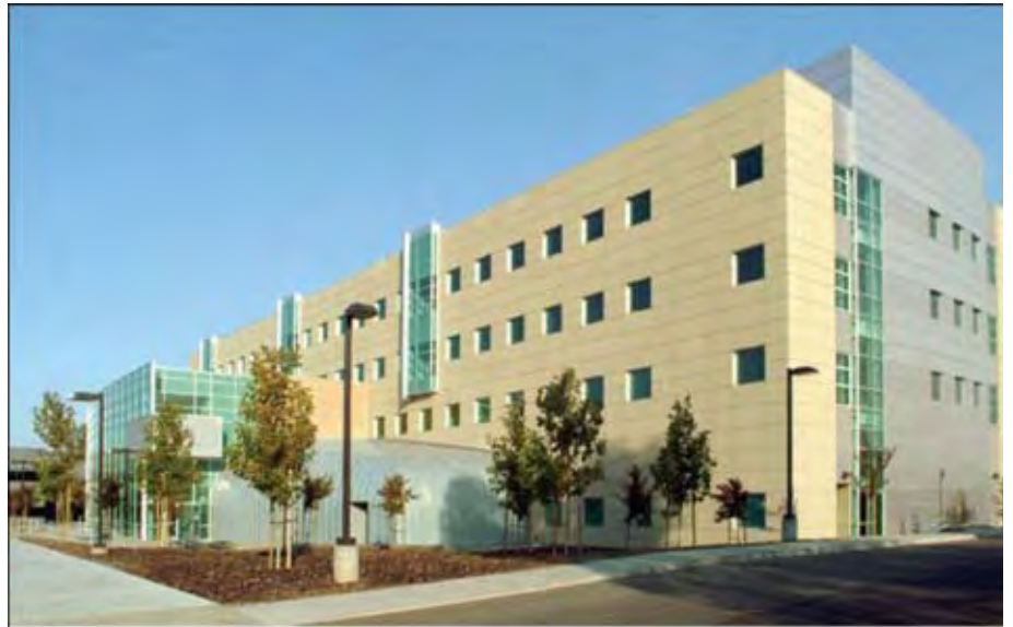
Figure 1. The TSF houses a total of 48,000 square feet of computer space with a projected load of 23 MW. The facility requires reliable electric power to ensure that the computations are not interrupted.
